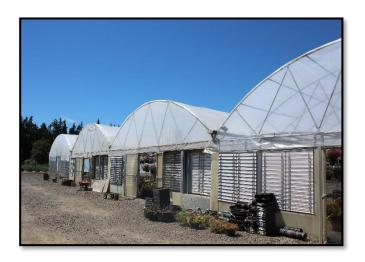
GK Machine's 9000 Series gutter-connected greenhouse design has superior airflow and temperature control and is suitable for multiple and varied vegetable crops, plants, and nursery crops. There are many ventilation options for GK Machine 9000 Series gutter-connected greenhouses, whether you are interested in natural ventilation or forced air cooling. The roof design maximizes condensation control.
